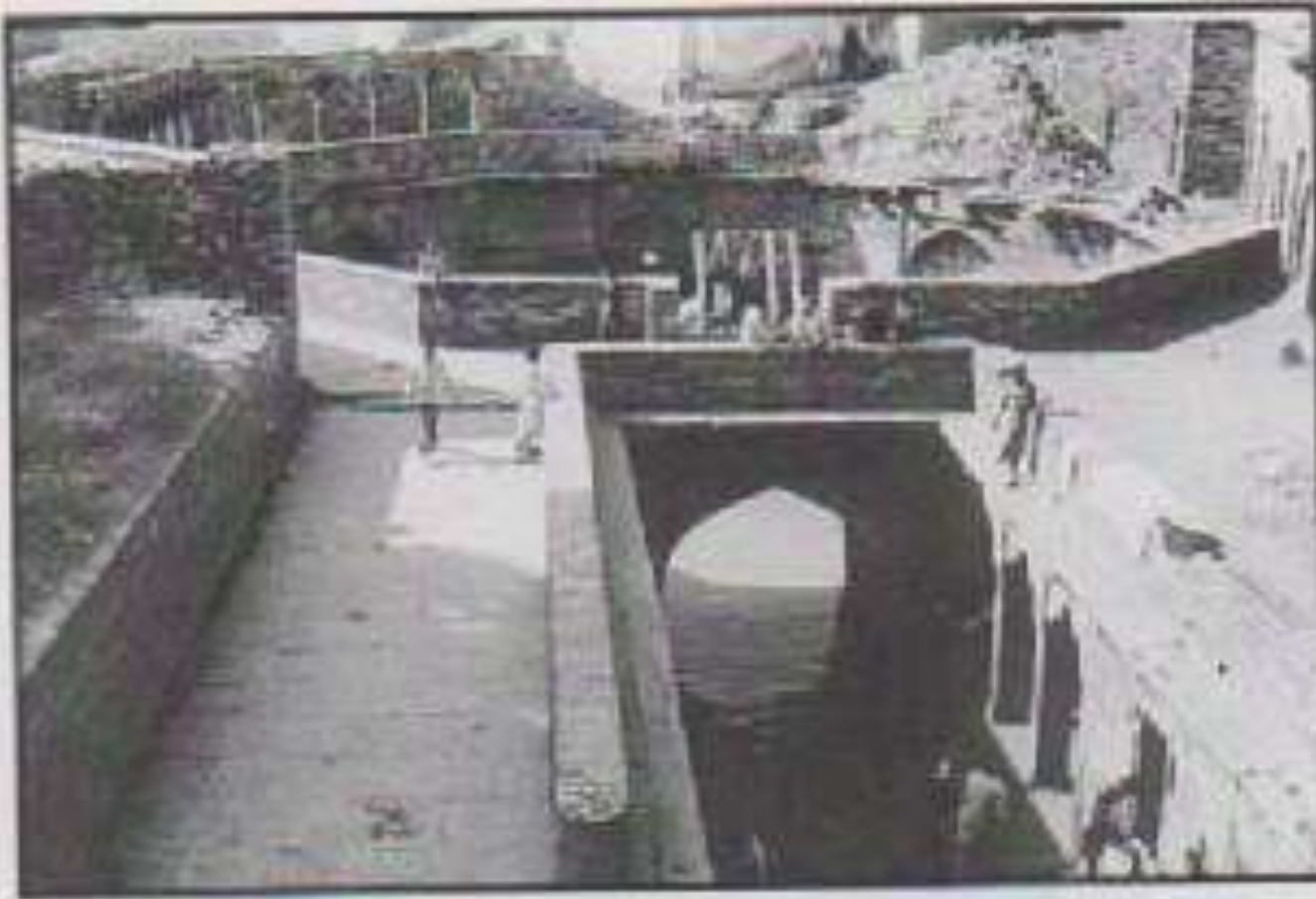
1. The Jhalra (Storage Tank) FPS
