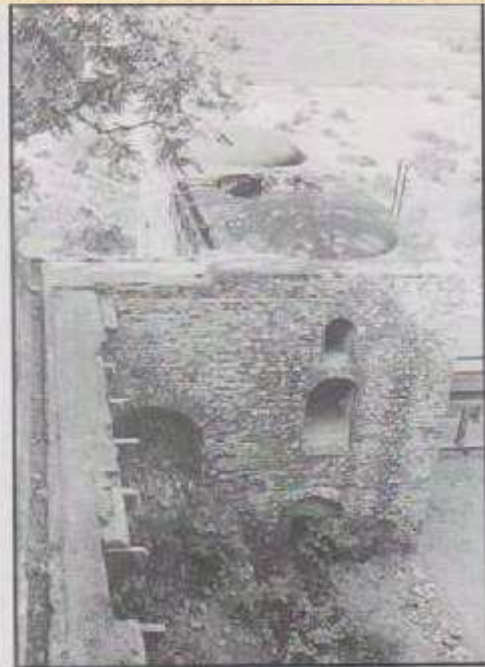
4. Overhead Channel near Sangin-Baoli
